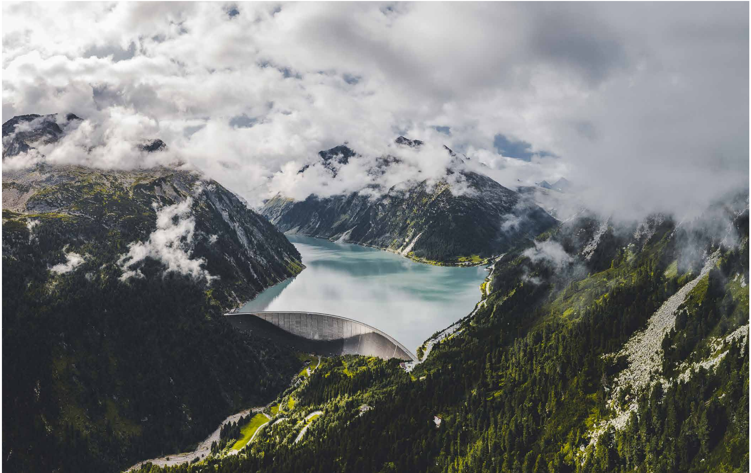
Thomas Holzmann - Schlegeis Speicher (Diga di Schlegeis), Zillertal, Mayrhofen (T)
